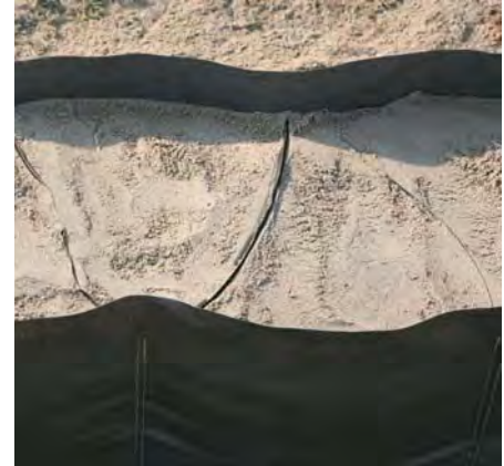
Fill Typar Matrix 3D cells with mulch, sand or other aggregate, depending on the application.
